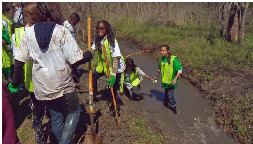
Students put on waders and dig trenches to lay PVC pipe.
